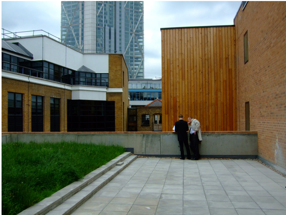
Larger of the two roof terraces, looking towards Scrutton Street
