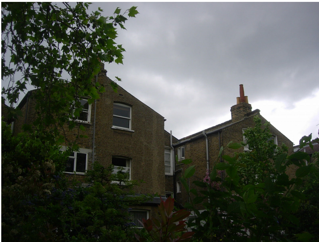
Figure 5: View north along the rear of the terrace
