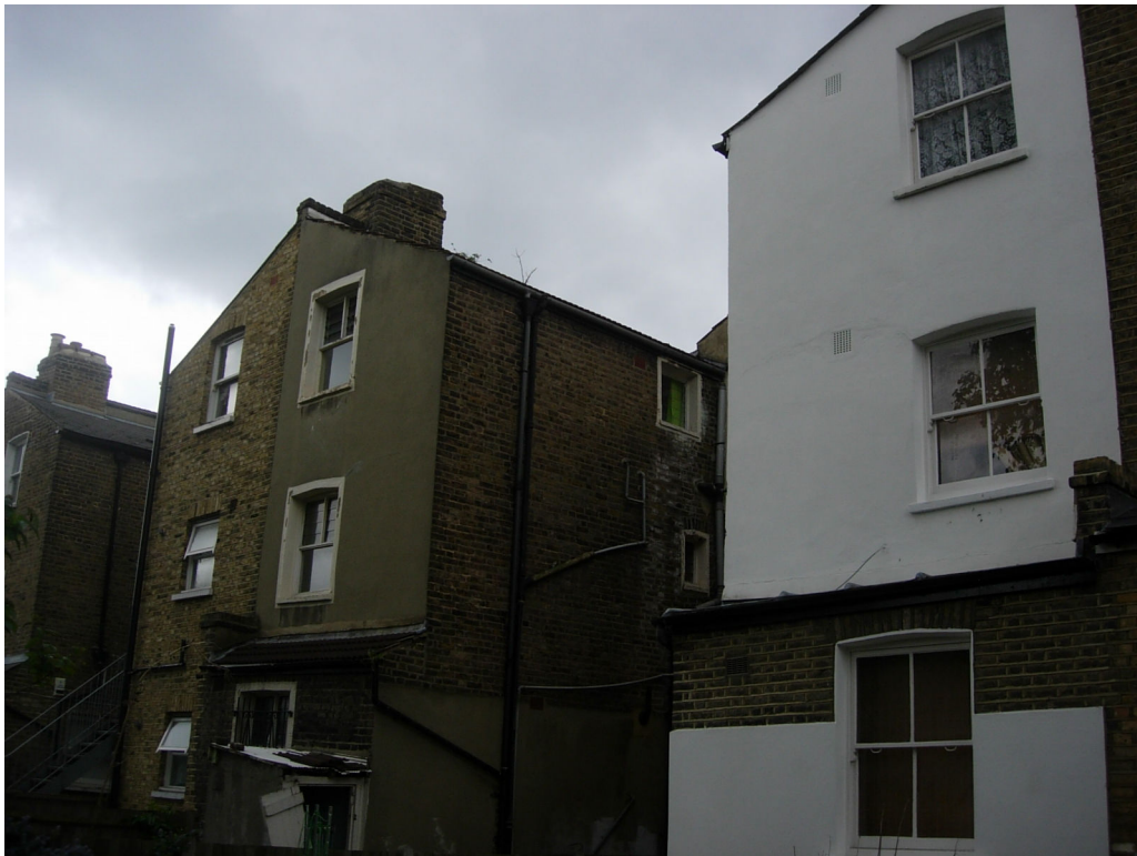
Figure 4: View south along the rear of the terrace
