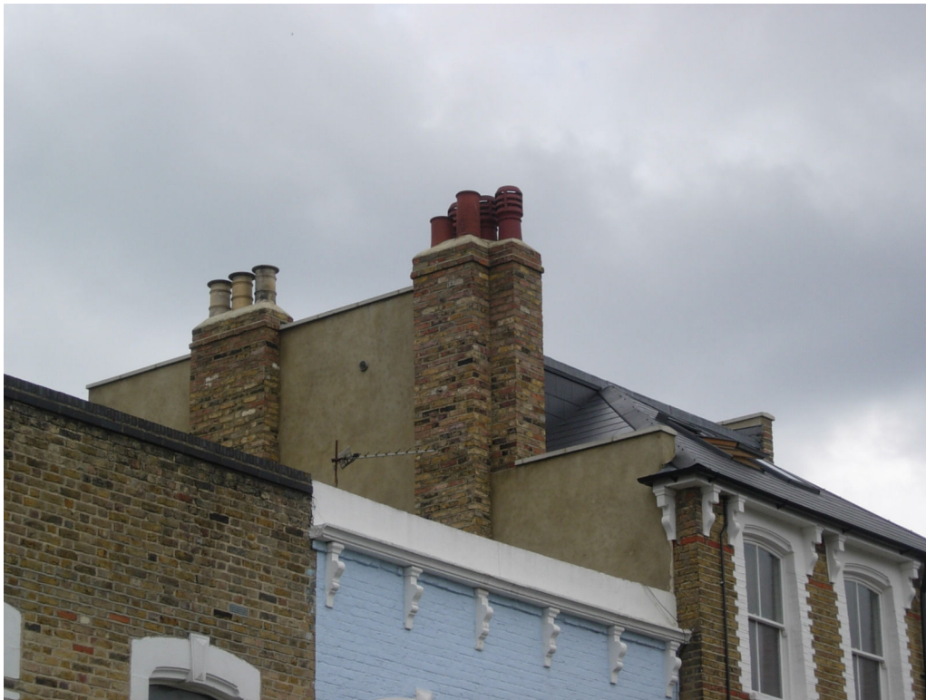
Figure 7: Roof extension viewed from the north
