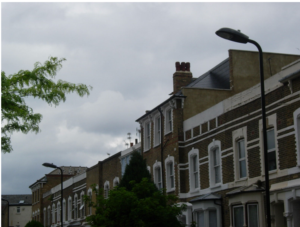
Figure 8: Roof extension viewed from the south
